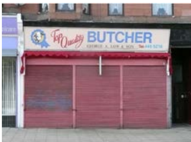
The solid roller shutters create a 'dead' shopfront when they are closed.
